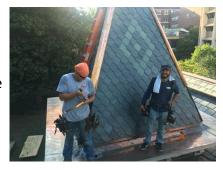
working with historical restorations is that a single roof on a house such as the one pictured can easily weight up to 60,000 pounds!" Rick added, "The sheer weight of each piece of slate makes the restoration dangerous and a little more complicated."
